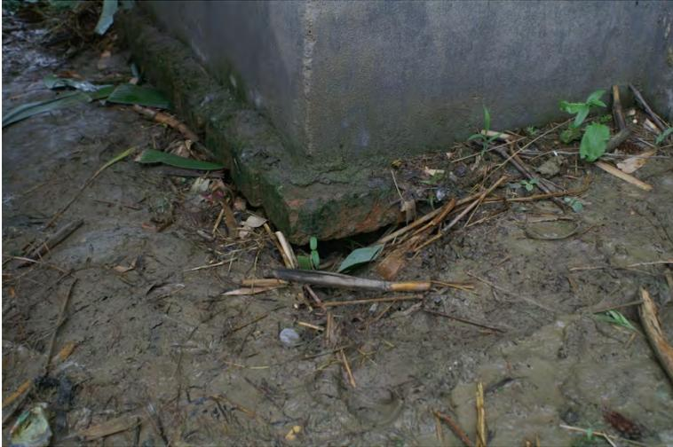
Figure 8: Erosion, exposing the brick base layer (Photo: Janis Koknevcis)
