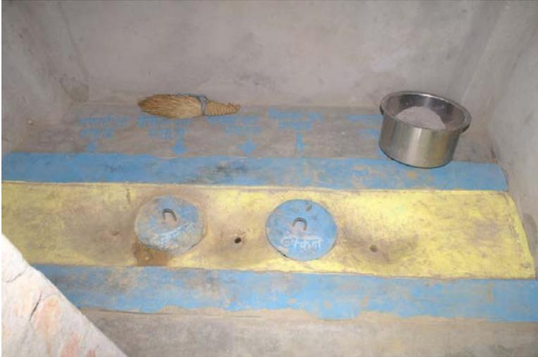
Figure 4: Inside of full brick and cement ecosan in Rupaliya (Photo: Janis Koknevics)
