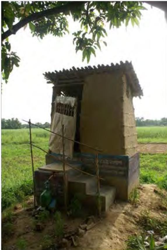
Figure 3: Ecosan toilet in Rupaliya, with mud, straw and bamboo super-structure (Photo: Janis Koknevics)
